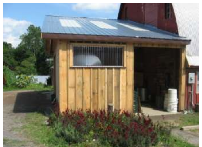
The Side View of our newly enclosed wash area
