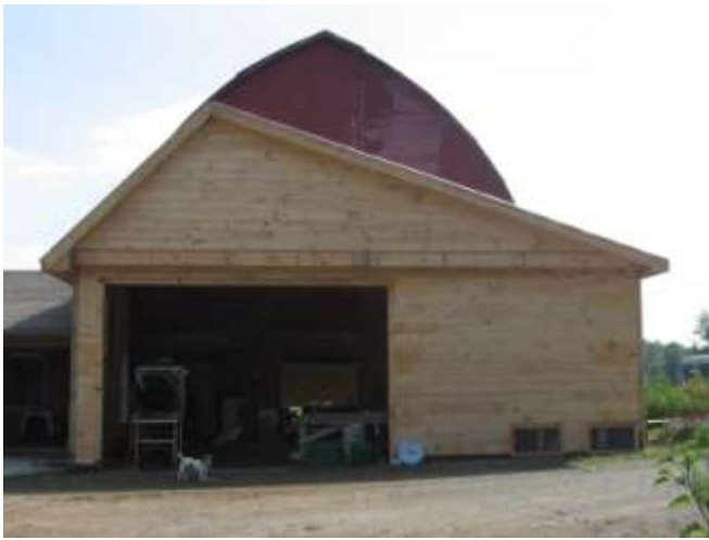
The Back view of the newly enclosed wash area
